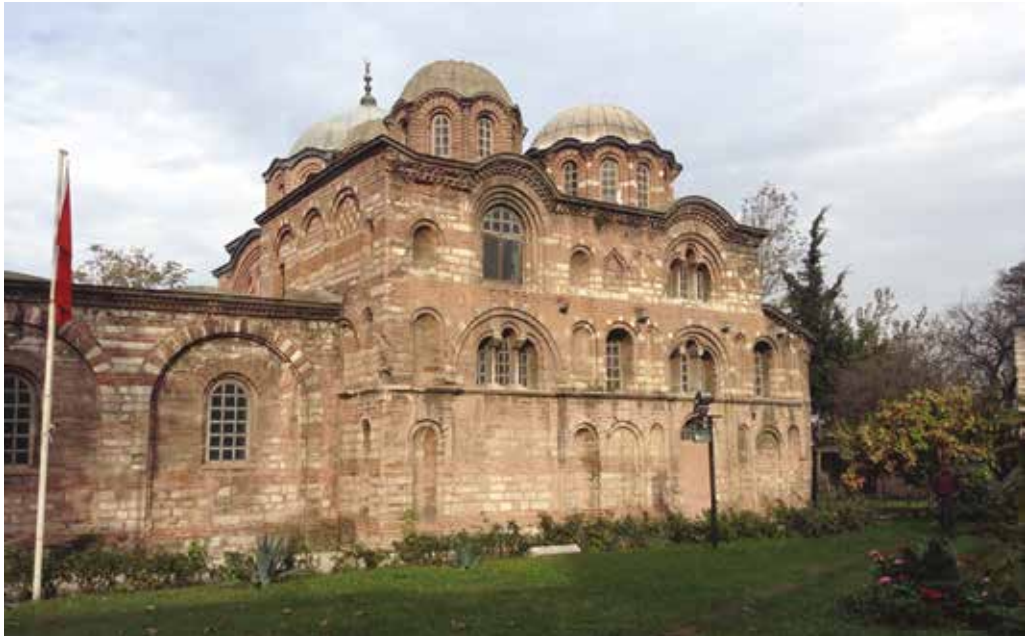
And this is a view of the exterior. Foto: Mariëtte Verhoeven
