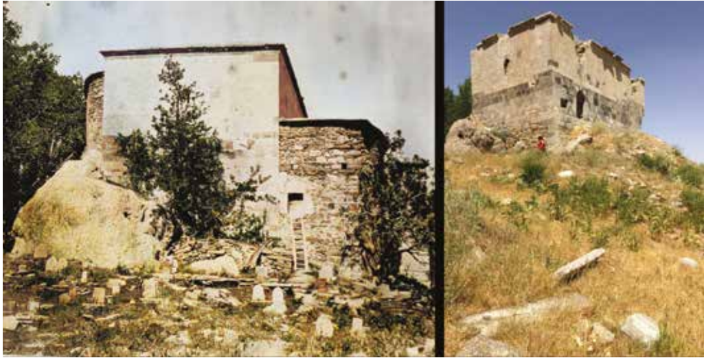
Figure 1. The exterior of the seventeenth-century patriarchal cathedral of St. Shallita at Qudshanis / Koçanis (Konak) before its abandonment in 1915 and in 2019. Photos : Mar Shimun Memorial Foundation, 1915 and Nicholas Al-Jeloo, 2019.
