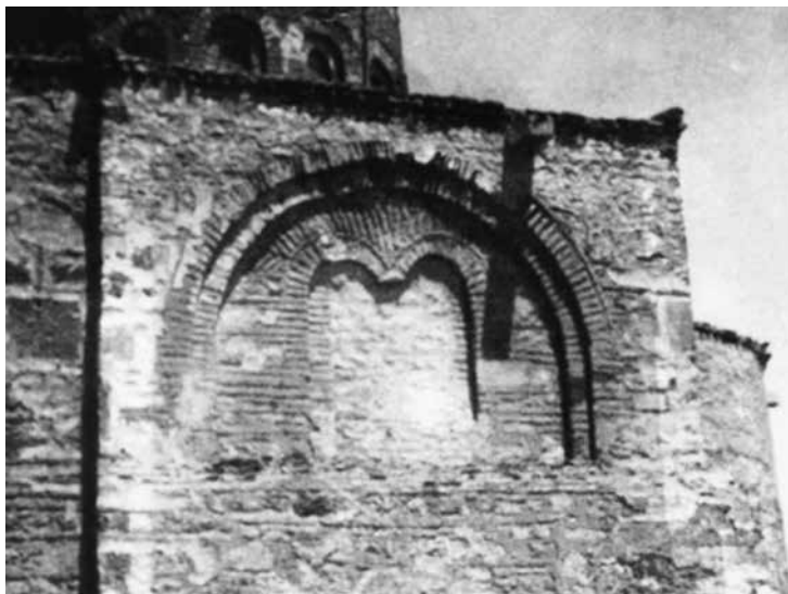
Figure 7. Details of fig. 4. The south tympanum and blocked window.
