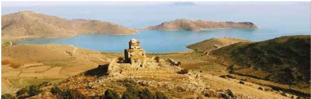
Figure 6: Van Gevaş Kantzag Surp Tovmas Monastery. The present state of the tenth to eleventh-century Monastery, located in the hamlet of Altınşaç Village in the Gevaş District of Van. Photo: M. Fatih Güden, 2019.
