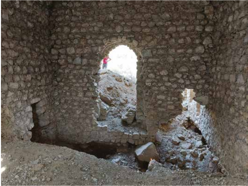
Figure 10. The interior of the church of St. George at Bayn-Ture / Bemtur (Çubuklu) in Şemdinli district, showing how the structure has been compromised because of illegal excavation by treasure hunters. Photo: Nicholas Al-Jeloo, 2020.
