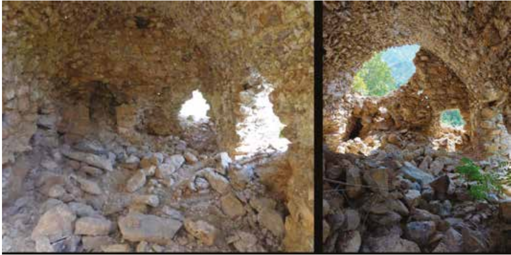
Figure 11. The interior of the St. Mamas church at the neighborhood of ‘Aqre / Akre (Akar) near Dağlica, showing signs of structural deterioration between 2015 and 2019. Photos: Nicholas Al-Jeloo, 2015, 2019.
