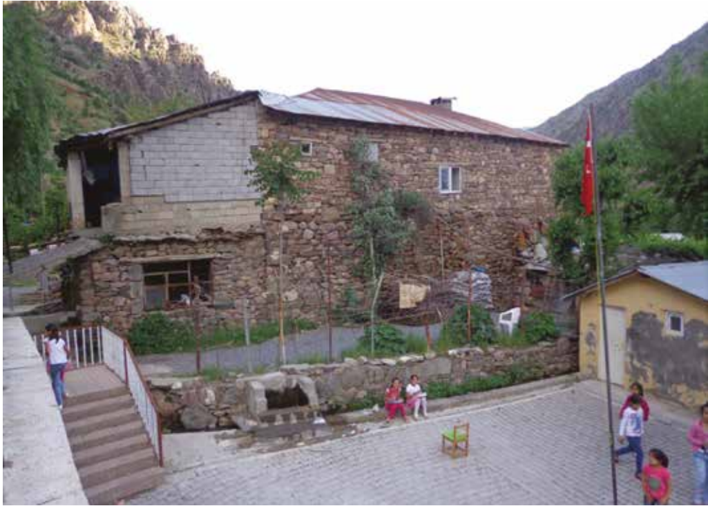
Figure 6. The church of St. Sava at Mazronka / Mezre in the area of Rumta / Rumtik (Geçimli). The upper level, which used to serve as a patriarchal residence, is now a private home, and the church on the ground level is now used for storage. Photo: Nicholas Al-Jeloo, 2015.
